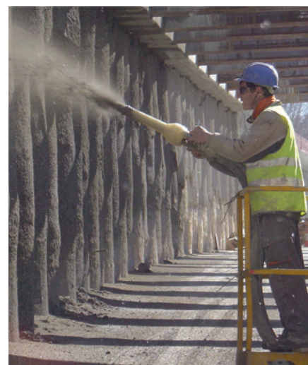
Fine concrete pumps like the P 715 are one of the most versatile of systems. You can use them for shotcrete ...
