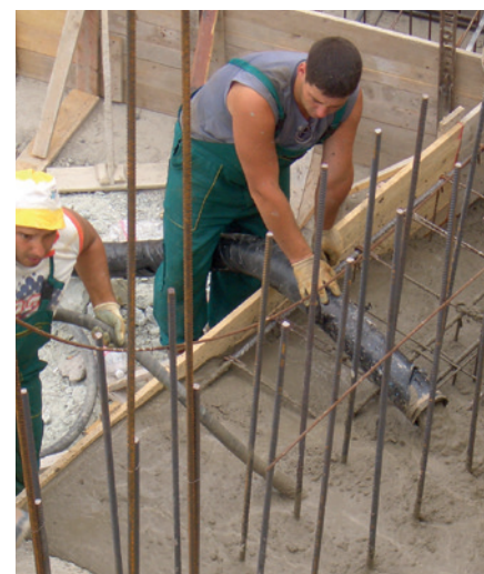
... or for pumping fine concrete of up to 16 mm. Because of the self-sealing and adjusting ring, you can even use them for liquid screed (right-hand picture).
